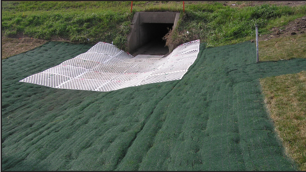
Figure 6.71 Transition mat as an alternative to rip rap. Source: Erosion Tech LLC
