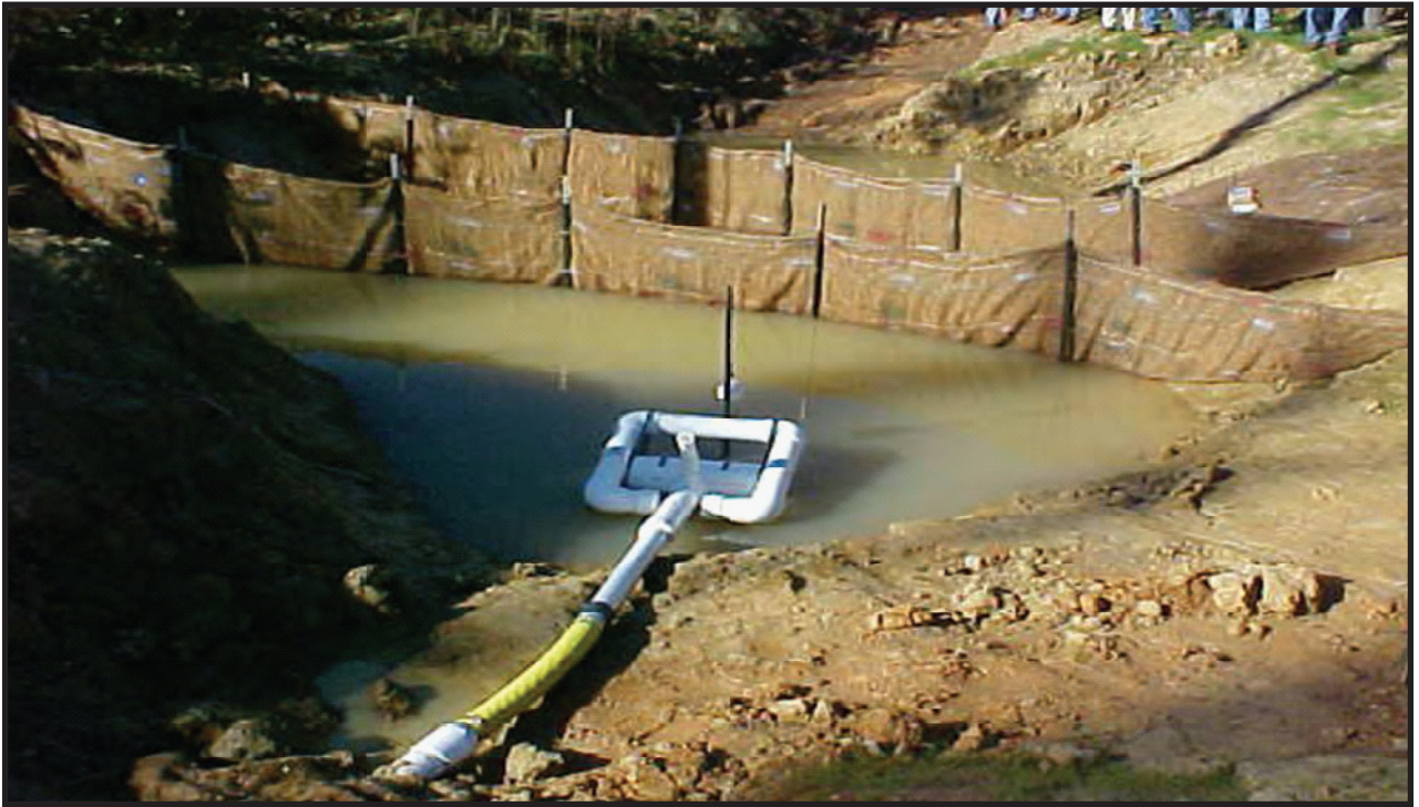
Figure 6.94 A skimmer that provides dewatering from the top of the sediment basin. Source: North Carolina Erosion and Sediment Control Planning and Design Manual .
