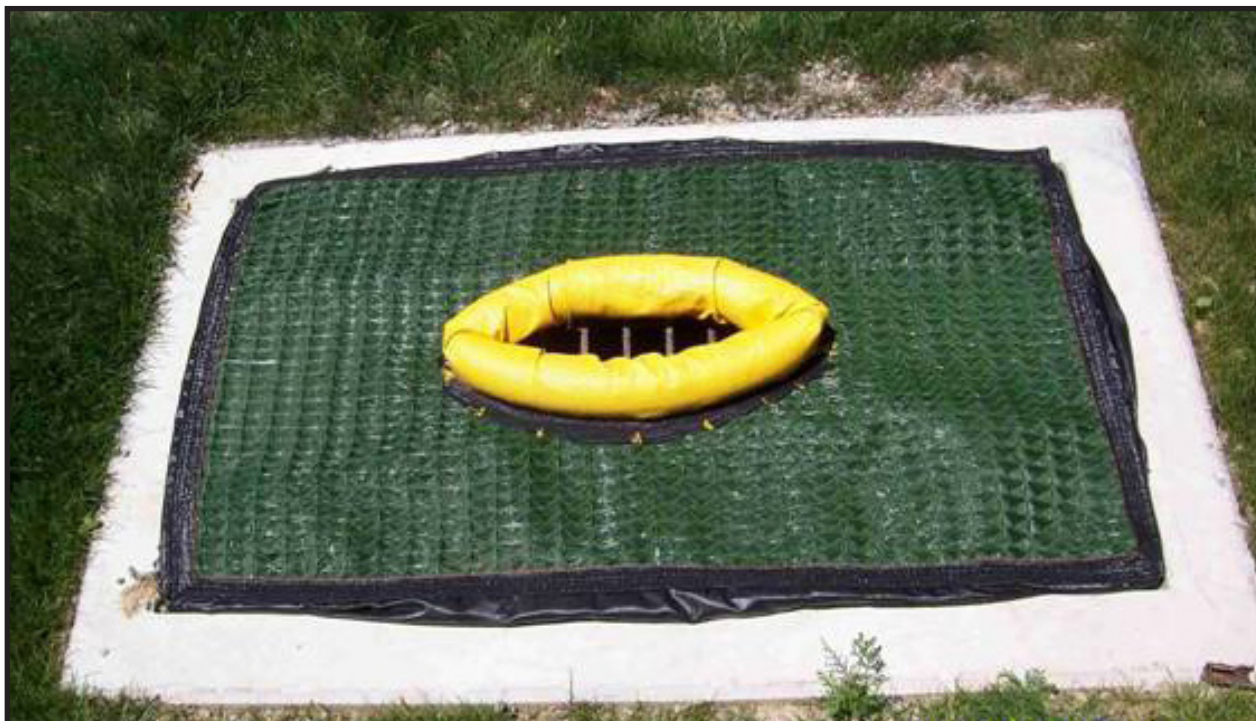
Figure 6.49 Inlet cover with opening for overflow.
