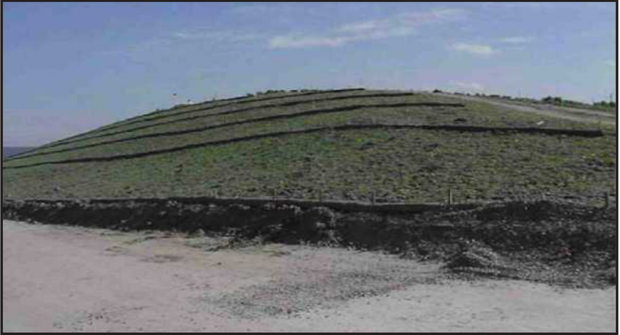
Figure 6.83 Wattles are used here as slope breaks to reduce the velocity of overland flow. Source: Missouri Department on Natural Resources Southwest Regional Office
