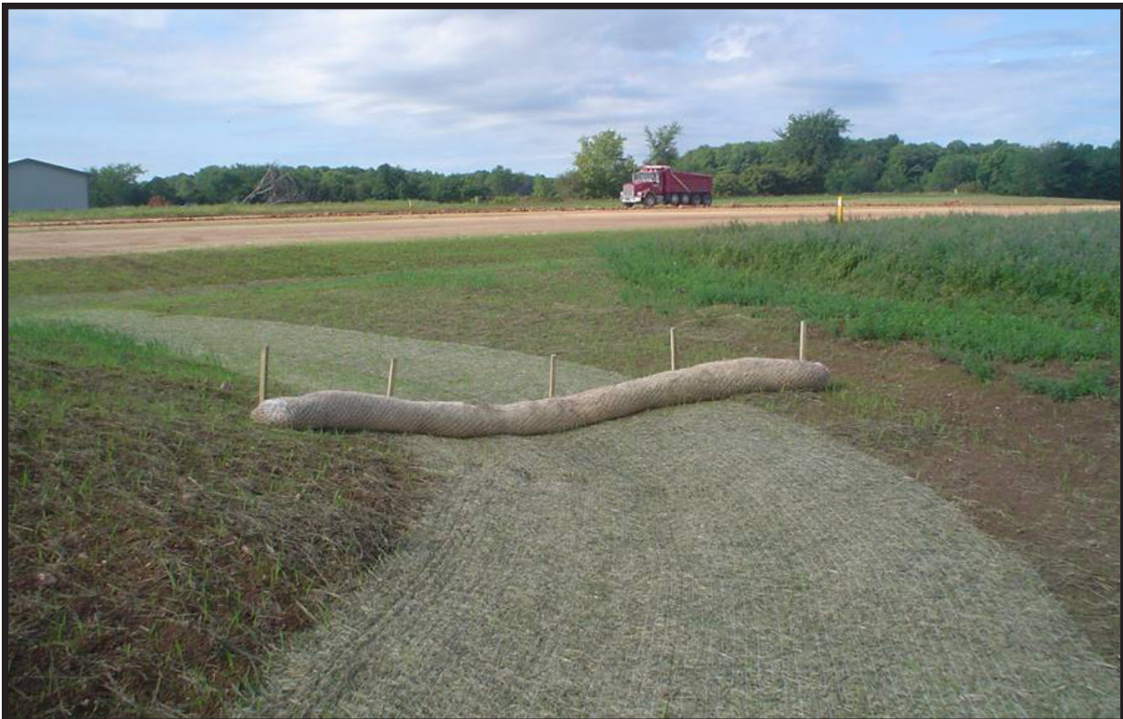
Figure 6.82 Wattle Ditch Check Source: American Excelsior
